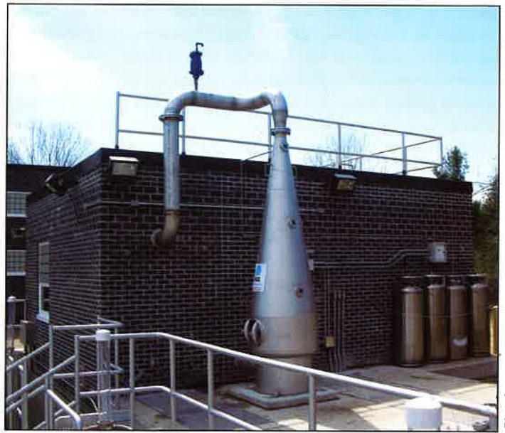
Superoxygenation system was installed here at Kennebunk, Maine for dissolved oxygen compliance of total maximum daily load.
