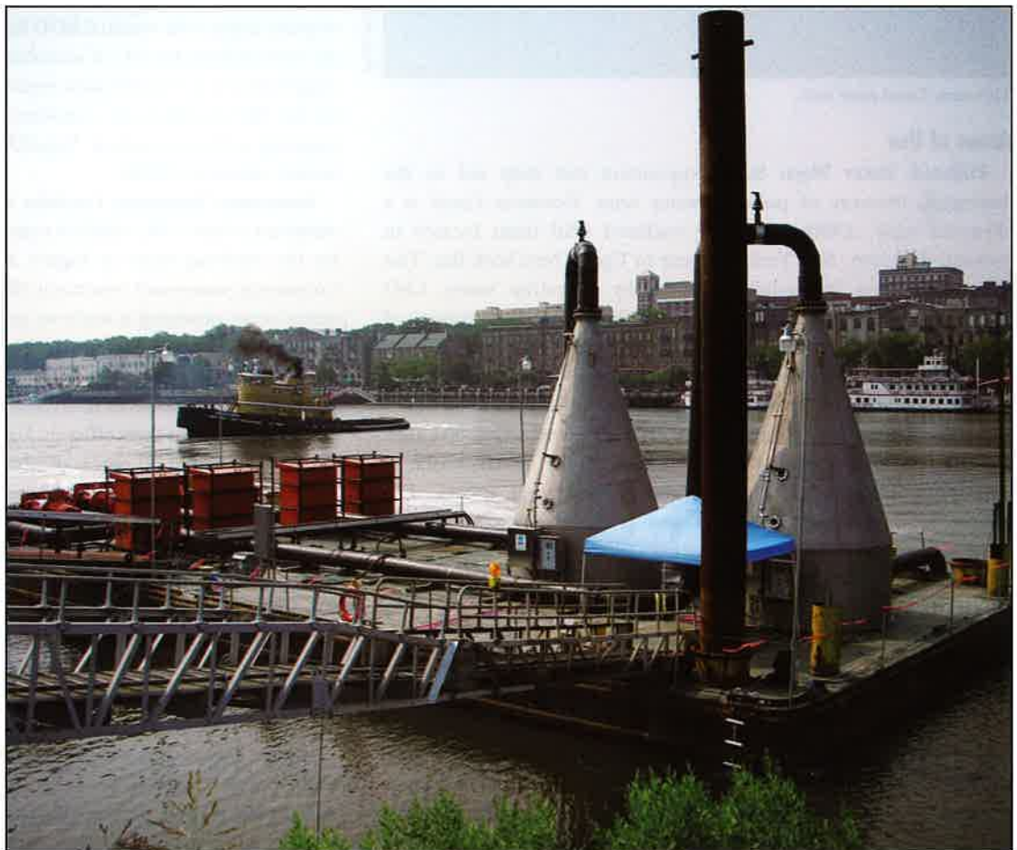
Superoxygenation was installed to correct dissolved oxygen after deepening of Savannah Harbor.
