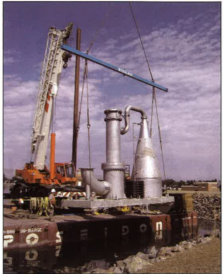
Superoxygenation was employed in the drinking water Marston Reservoir in Denver, Colorado
