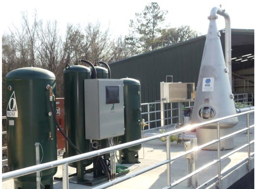
ECO<sub>2</sub> System and PSA Oxygen Generator
