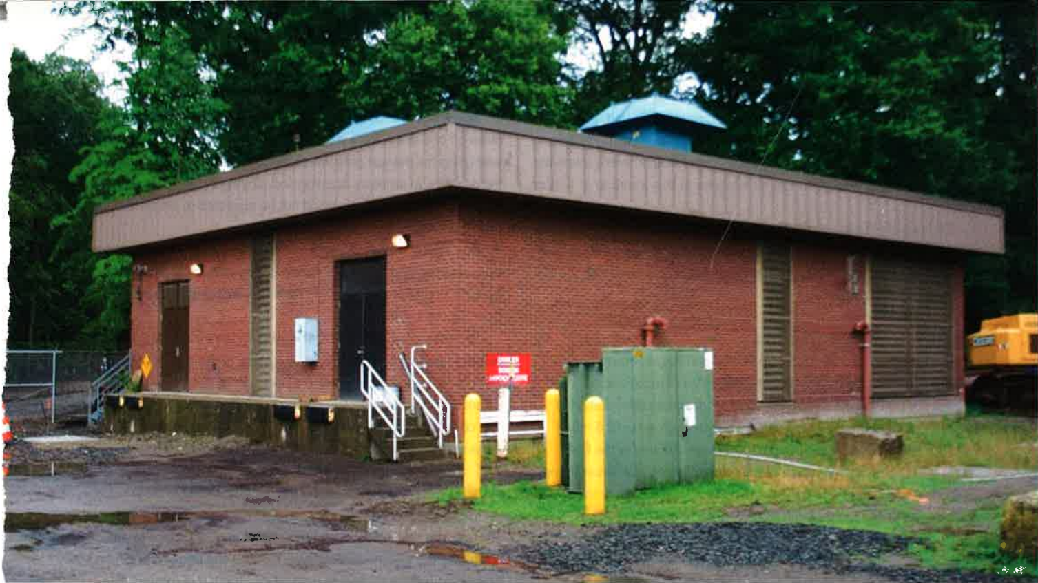
The Gulf Pond Pump Station in Milford, Conn., discharges into two force mains. Before upgrades and fixes, these force mains were the source of high levels of hydrogen sulfide, which led to odor and corrosion problems throughout the downstream system. Charlie Smith/AECOM
