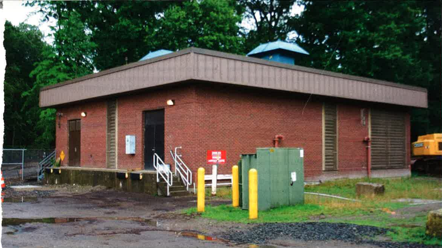
The Gulf Pond Pump Station in Milford, Conn., discharges into two force mains. Before upgrades and fixes, these force mains were the source of high levels of hydrogen sulfide, which led to odor and corrosion problems throughout the downstream system. Charlie Smith/AECOM
