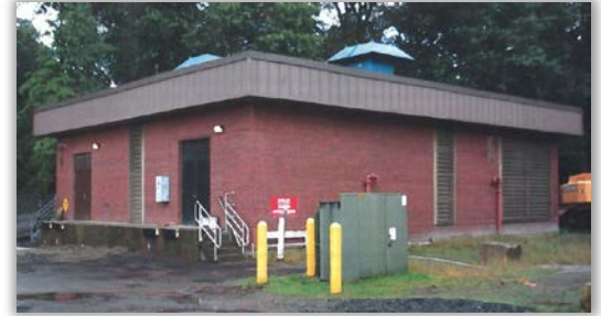
Gulf Pond Pump Station Building
