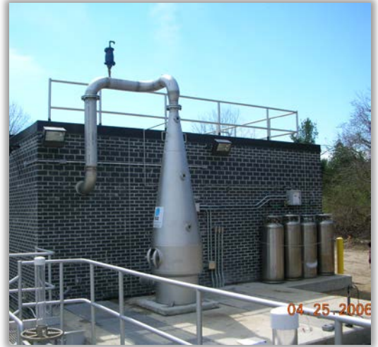
Installation of ECO 2 system at the Kennebunk WWTP Effluent
