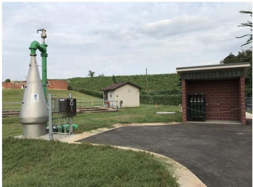
ECO<sub>2</sub> System and 12 Pack of Oxygen Cylinders
